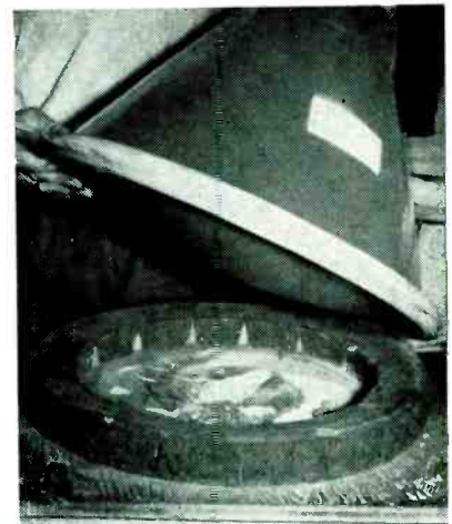
Felt-padded ring supports metal-wall tube while plastic dress is put on
